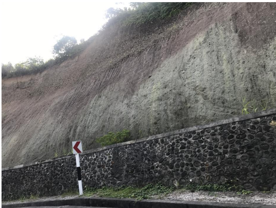
Figure 5. Slope protection structure at Barangay Naagtan
